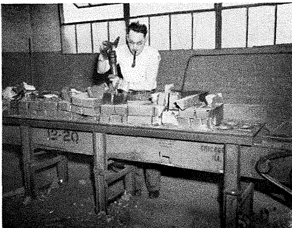
FRED BISHOP uses a small air hammer to break up the mold around an aluminum casting. The castings are then vibrated to remove molding sand which is removed by a moving belt.
